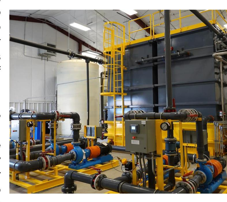
We design, manufacture, supply and commission treatment plants for various types of industrial effluents like textile, chemical, distillery, paper and pulp, aluminum by combining physicochemical treatment followed by tertiary treatment for the removal of inorganic solids, heavy metals and finer suspended solids.
